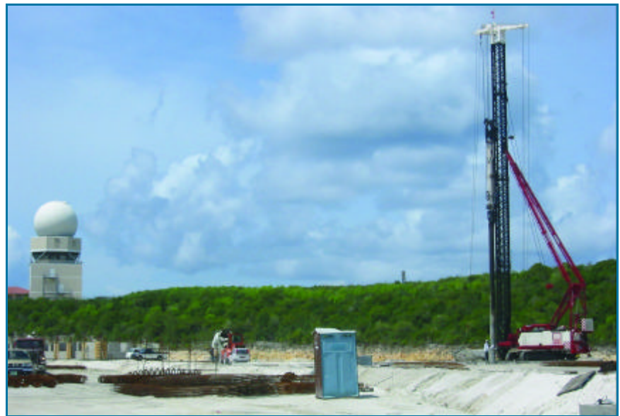
West side view of the expansion works.
