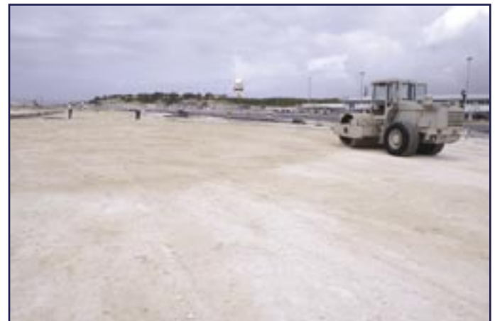
The project site
